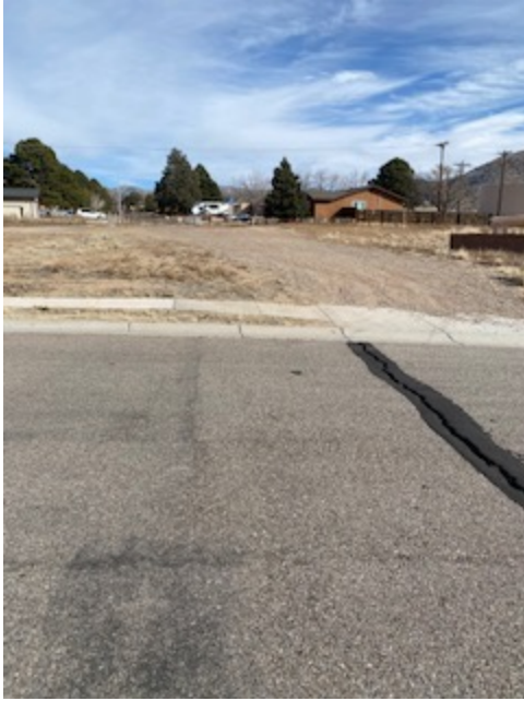
View of Rio Arriba Ave Exit gate looking east
